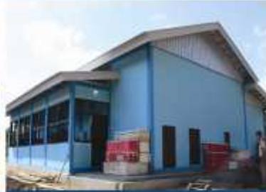
Coldstorage 50 Ton (PPI Daruba)
